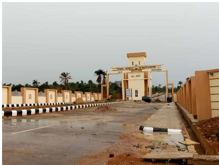
Overview of the Construction of Perimeter fence and Security Gatehouse
